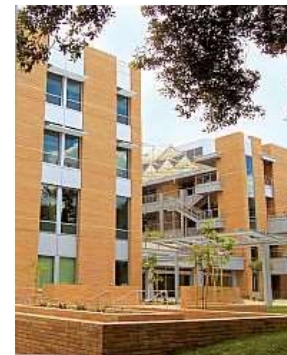
UCR Engineering Building
